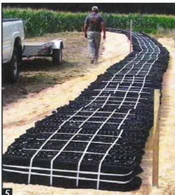
Fig. 4. GSF system installation before backfilling.
