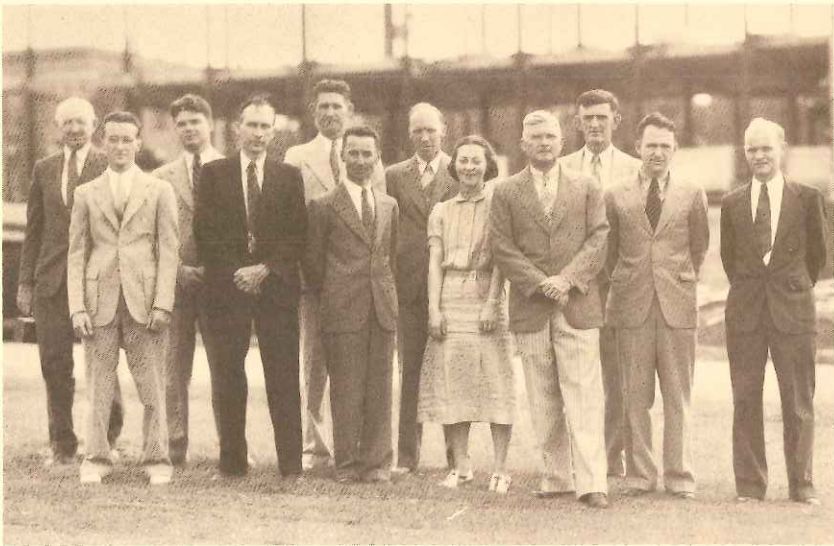
Agricultural Engineering faculty and staff standing in front of the Agricultural Engineering Building under construction, 1938.
