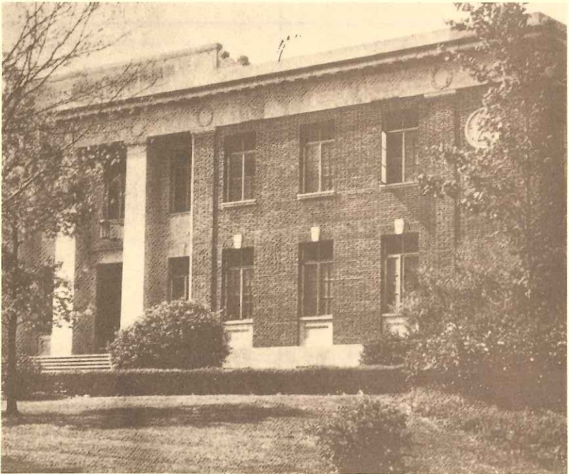
Agricultural Engineering Building
